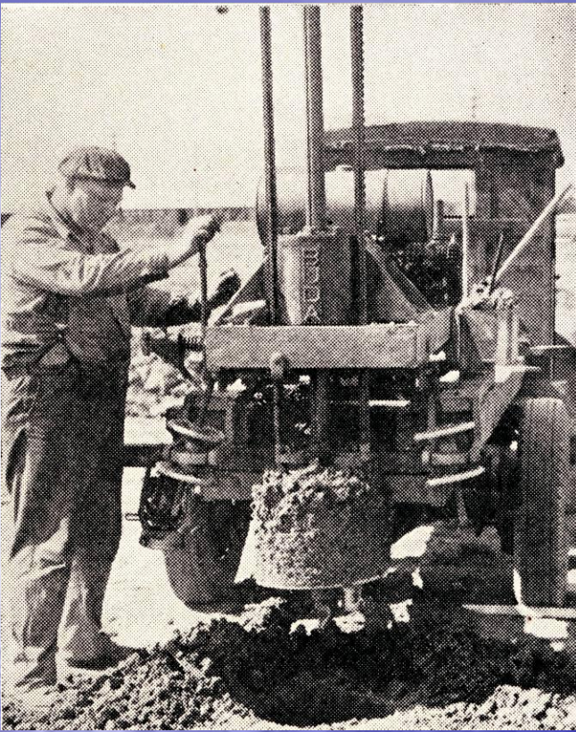
Gas powered spud drill – early 1920's
